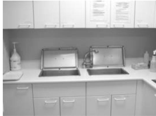
Instruments are cleaned in the ultrasonic cleaners
